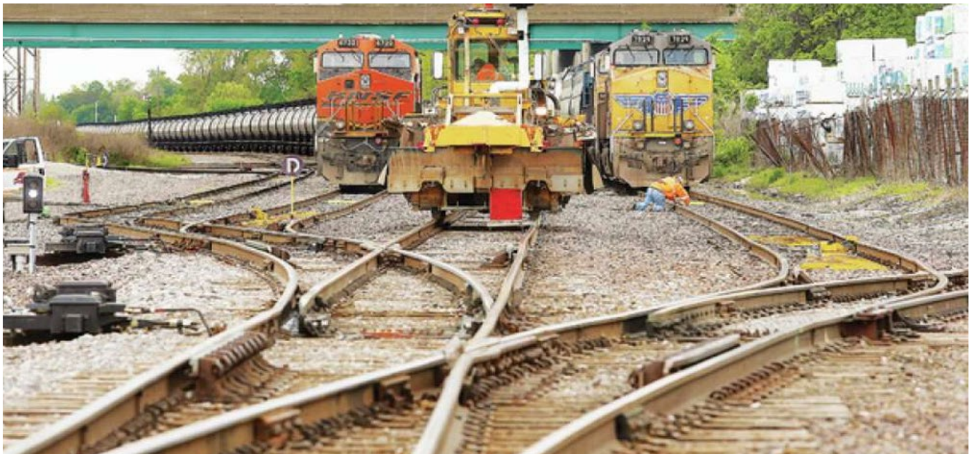
An average of 66 trains pass through the Lenox Tower interlock, which is located at the intersection of four railroads: Union Pacific, Canadian Pacific Kansas City, Norfolk Southern, and Alton & Southern. Movements were restricted by diverging turnouts and a specialty track switch known as a single slip switch.
