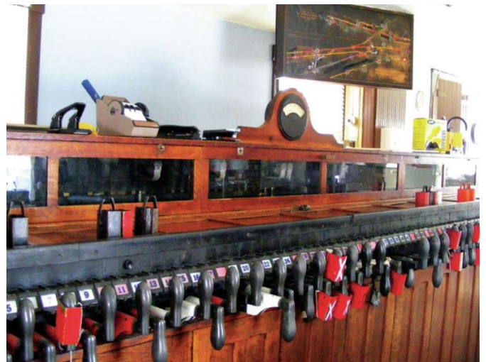
The 80-lever G pistol-grip electric interlocking machine was housed in a large wooden console. A track model board above the console showed the 80 switch locations on each of the railroad tracks.
