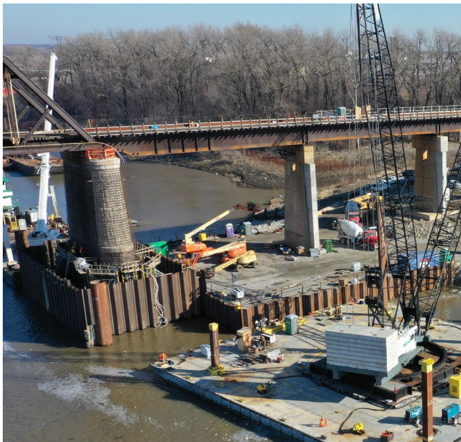
Constructing the bridge pilings
