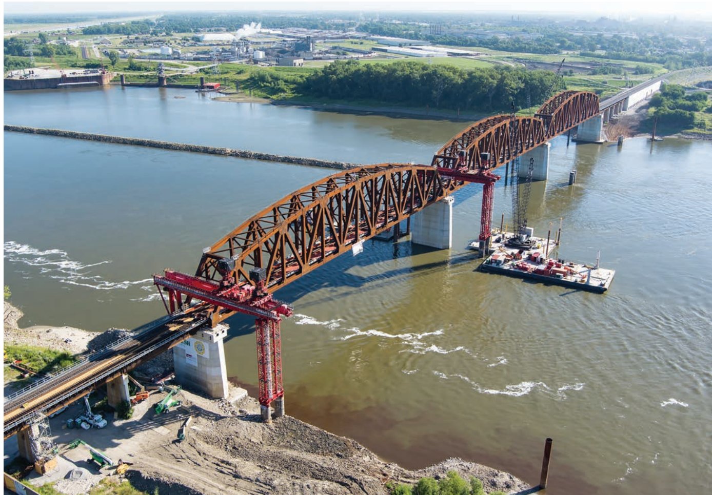
All Merchants Bridge photos courtesy of Walsh Construction and Trey Cambern Photography
