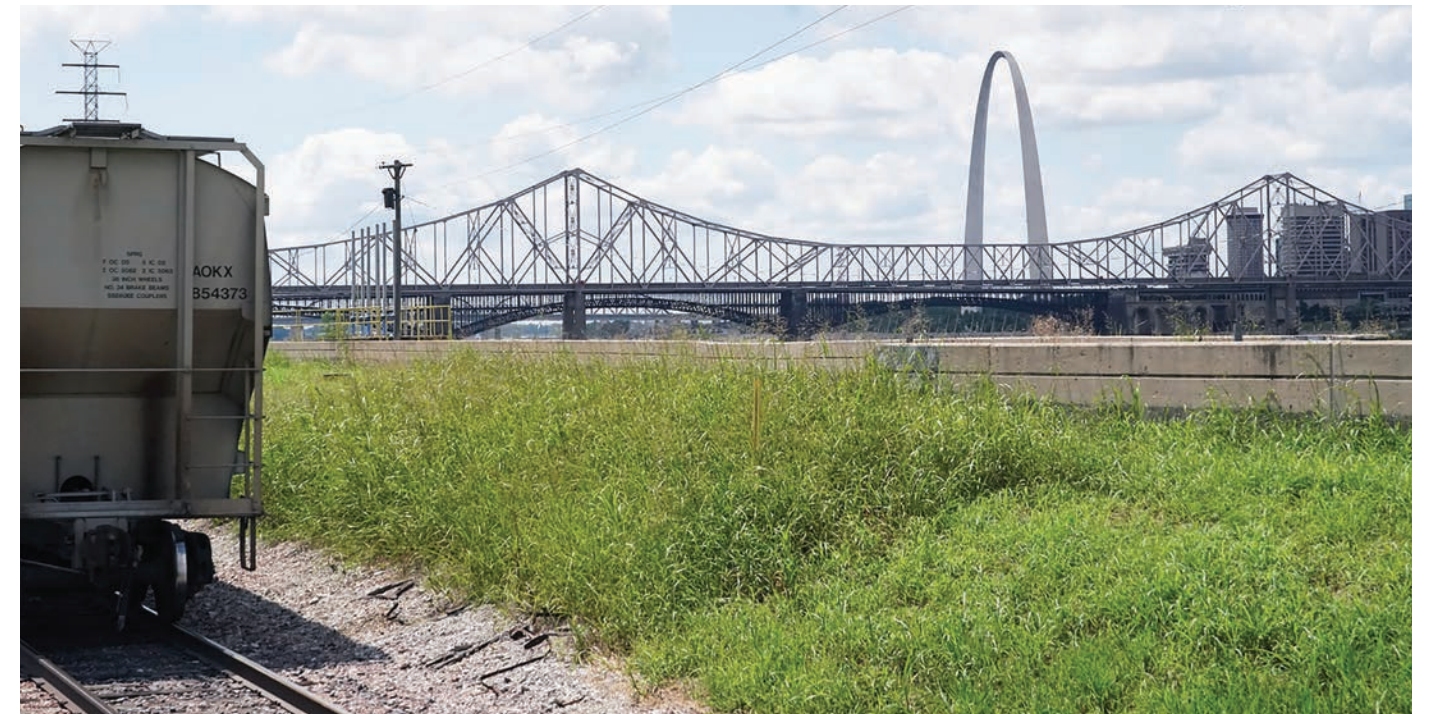
Martin Luther King three-lane bridge just north of downtown St. Louis with direct access to major highways
