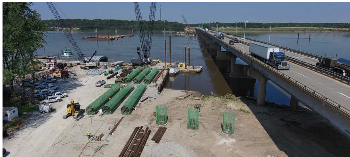
Chain of Rocks Canal bridge replacement
