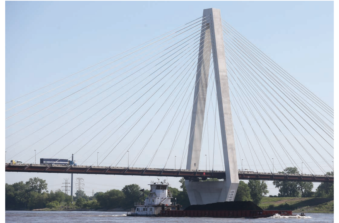
The Stan Musial Veterans Memorial Bridge across the Mississippi River, the finishing line for the I-70 Improvements.
