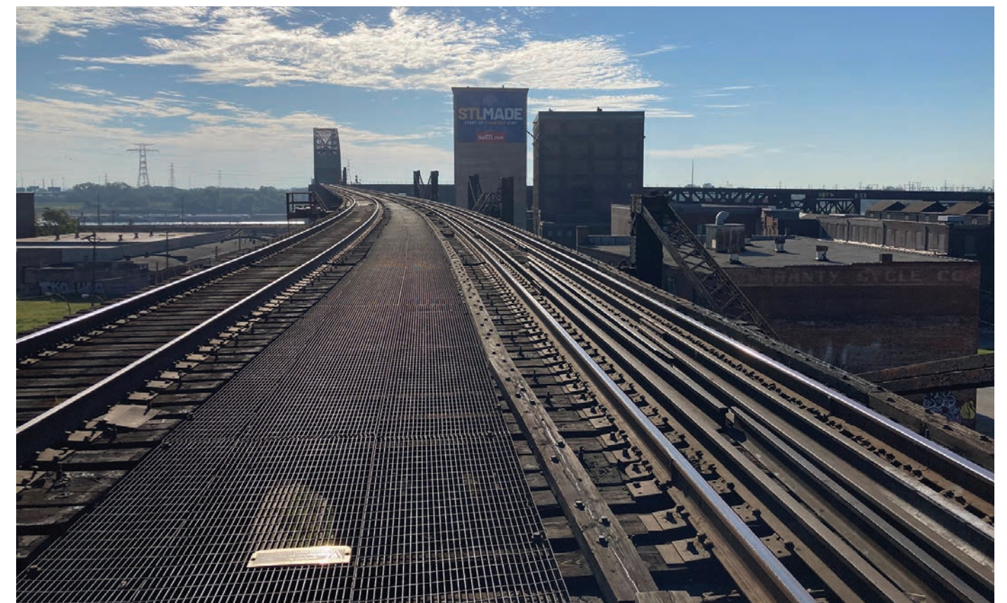
MacArthur Bridge just south of downtown St. Louis
