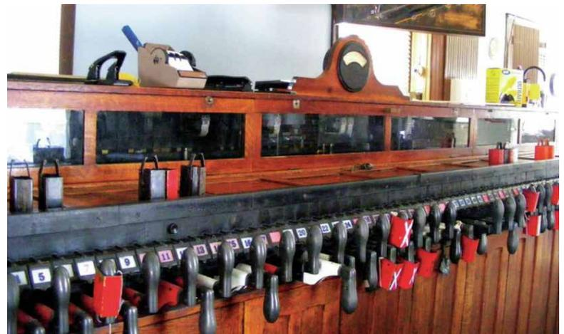
**Right (Top):** The Lenox Tower’s interior housed the operator’s office and the interlocking equipment, which consisted of the interlocking machine and track model board. The Lenox Tower was one of the last three manually operated interlocking plants in the St. Louis Area in Illinois.
